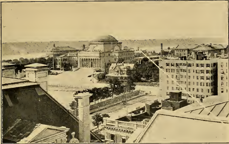
LOOKING NORTHWARD, NEAR THE UPPER END OF THE NEW HARLEM LINE.
